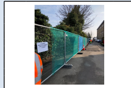
21/2/18 - The roadway is fenced off so vegetation cut back can occur
