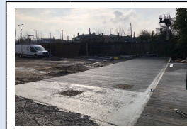
21/2/18 - External slabs to the service yard being poured
