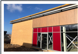
5/1/18 - The Costa Cladding being installed to Unit 3
