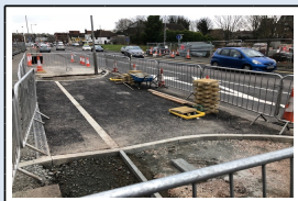
3/1/18 - The entrance being constructed to St. Michael's Road Car Park
