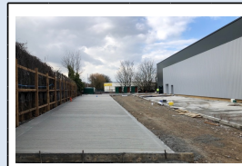
7/3/18 - Only one concrete slab remaining for the service yard area
