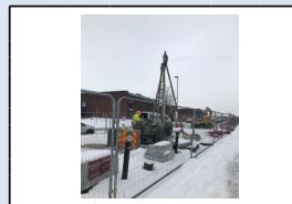
1/3/18 - Site investigation works being undertaken for contamination
