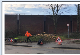
5/2/18 - Tree felling on the site of the new multi-storey car park
