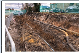
6/3/18 - The shrubbery bank is removed and an uncharted water pipe encountered
