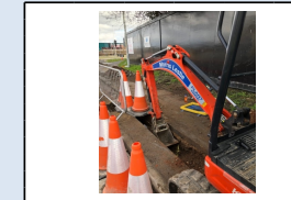
6/3/18 - Ducting being installed in Milton Rd for the controlled crossing
