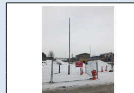
1/3/18 - Lighting Columns installed in St. Michael's Road
