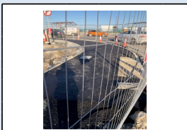
17/1/18 - The new footway being asphalted
