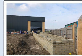
21/2/18 - Construction of the pedestrian ramp off Eurolink Way
