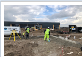
7/3/18 - Kerbing being laid to form the car parking areas
