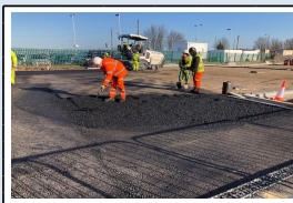
17/1/18 - The first day of asphaltting to St. Michael's Road car park
