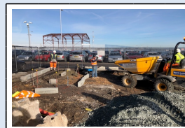
8/2/18 - Works start on the breakthrough area
