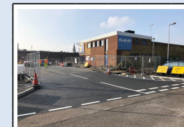
21/2/18 - The completed breakthrough area
