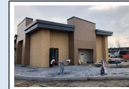
21/2/18 - Hard Landscaping being installed around Unit 3 (Costa)
