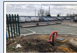
13/2/18 - Formation installed and compacted for the breakthrough area
