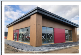
7/3/18 - Blockwork footpath and Cladding now substantially complete to Costa
