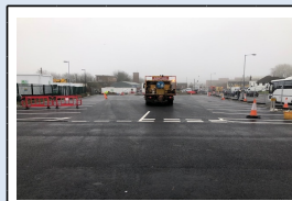
26/1/18 - Road marking being installed in St. Michael's Road car park
