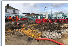
6/3/18 - Ducting for electrical cables and manhole covers start to be installed
