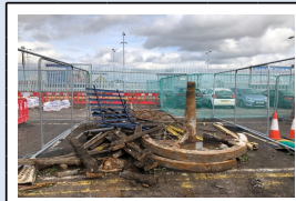
6/3/18 - Erith uncover an unknown circular metal structure encased in concrete
