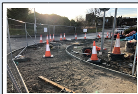
10/1/18 - The new footway being constructed in St. Michael's Road
