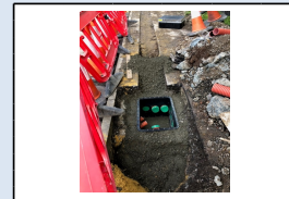
8/3/18 - Duct pit installed in Milton Road
