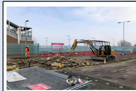
21/2/18 - The raised concrete slabbed area is broken up
