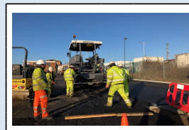
19/1/18 - Final day of asphaltting to St. Michael's Road car park
