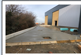
8/2/18 - External concrete slabs being poured to the service area
